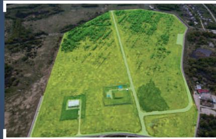
Rapid utility hookup
